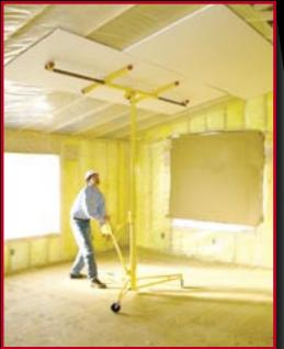
trunk of your vehicle for easy transport to your next job site. The tripod base folds to allow the assembled unit to pass through doorways. The PANELLIFT® is made in the USA using all-steel construction to handle commercial work loads.
