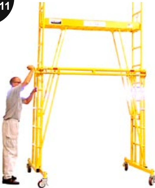
Insert the second set of rails in the top of the first.
